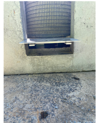
Field joint plate in position
